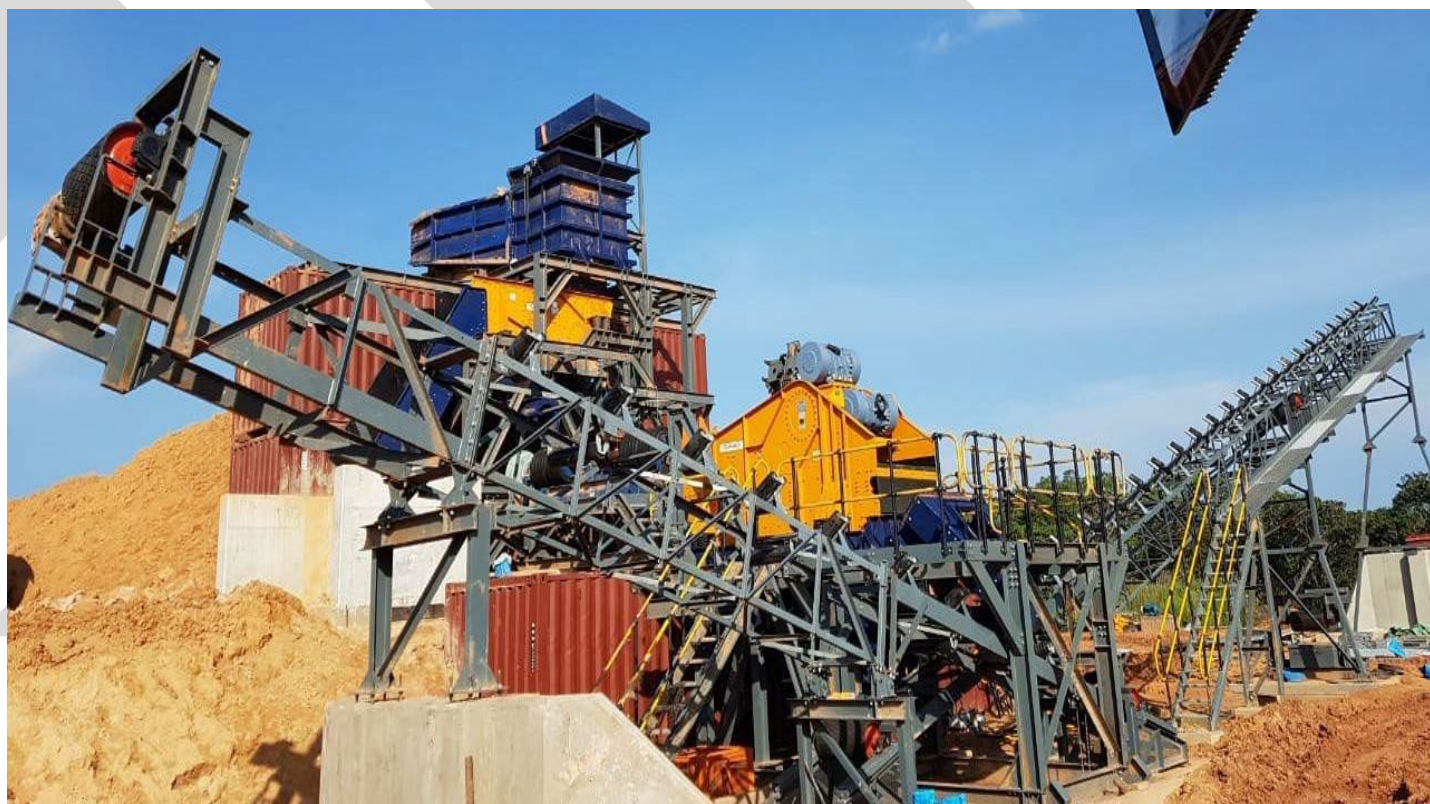
Wet-front end module with containers installation, Lucapa diamonds, Angola
