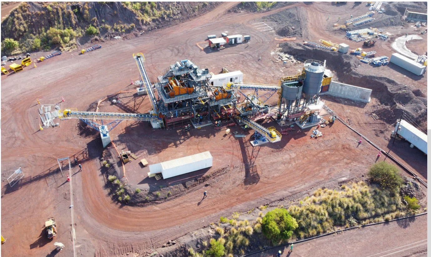
160 tph Iron ore super high DMS plant, GravMax, Northern Cape, South Africa
