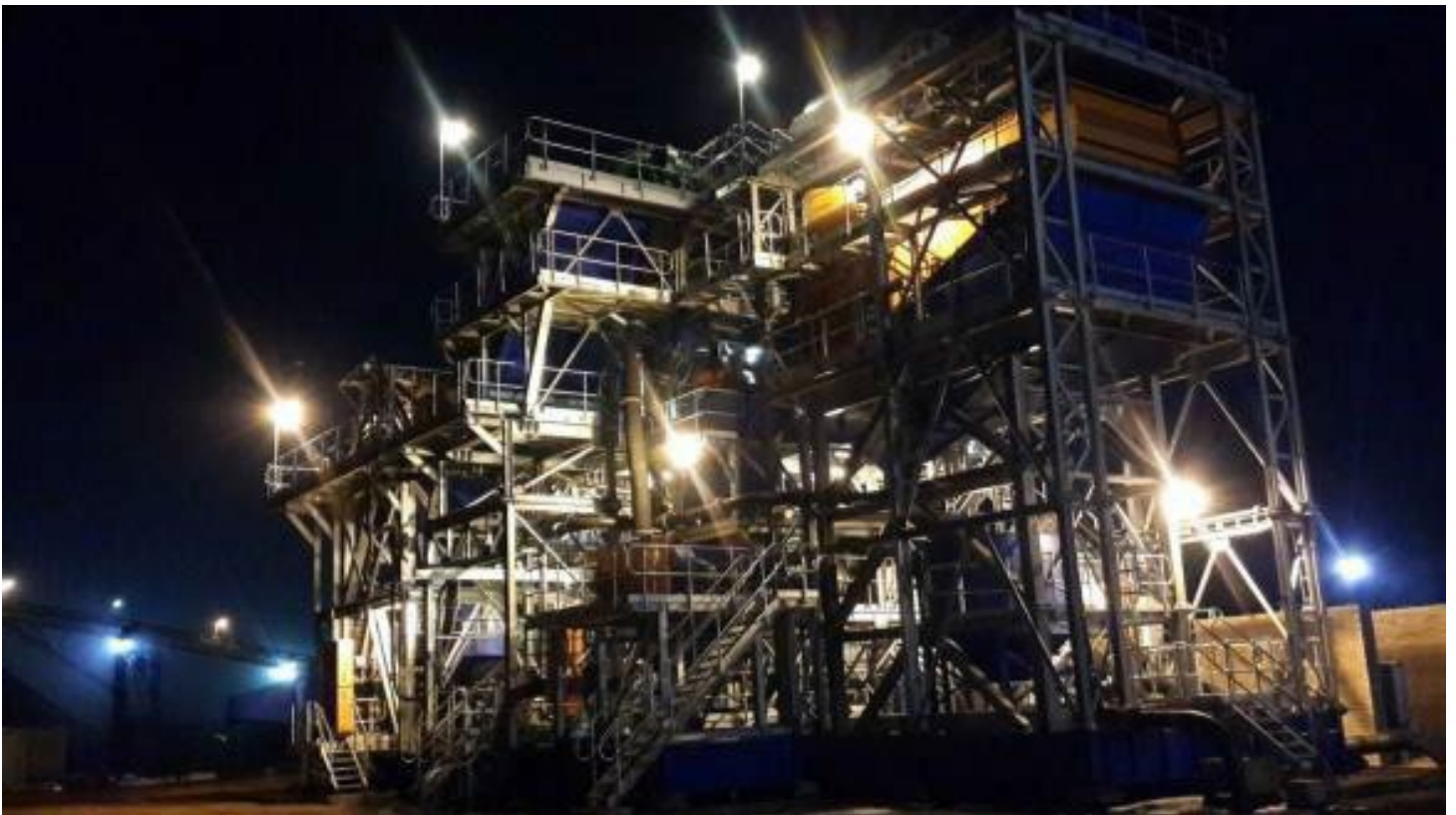
450 tons per hour coal DMS trial assembly at Consulmet fabrication works and completed installation Stuart Coal, Delmas, South Africa
