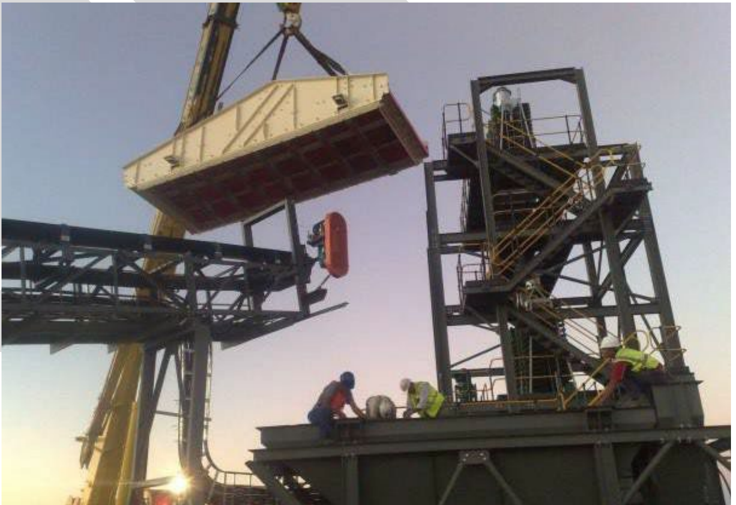
Screen installation at mineral processing plant satellite chrome, Rustenburg, South Africa
