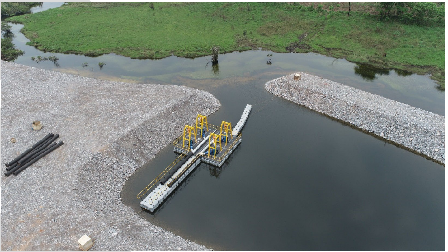
Floating barge pump system, Angola
